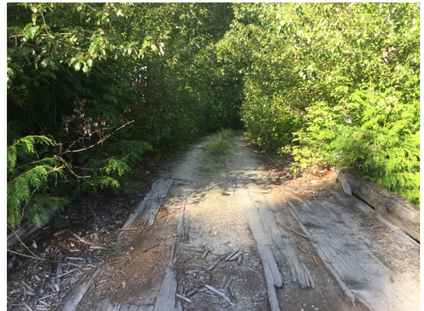
Left Approach Facing Away From Bridge
