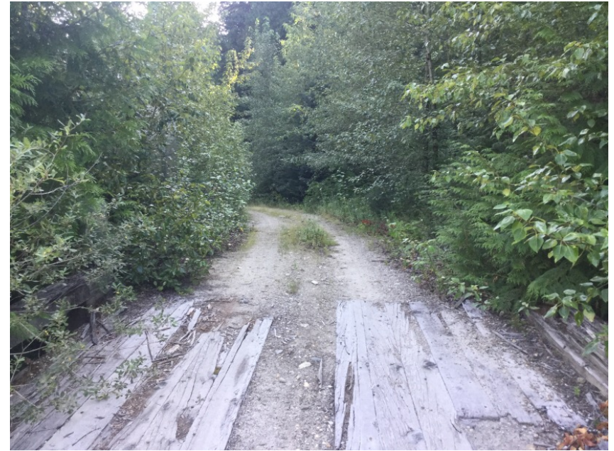
Right Approach Facing Away From Bridge
