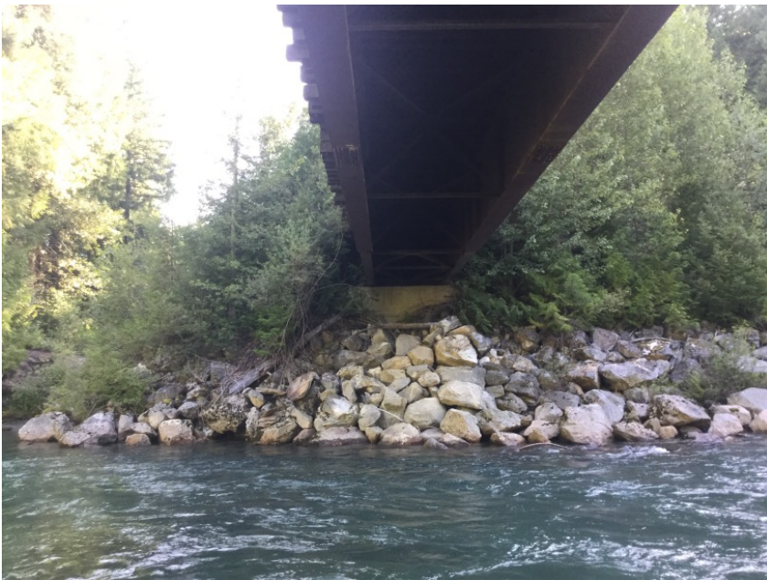
Right Bank Abutment
