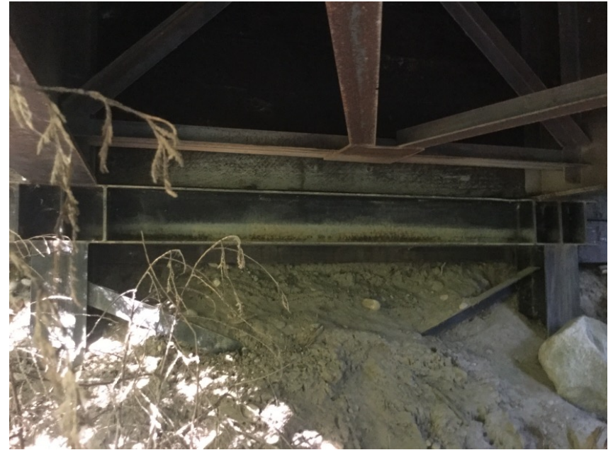
Left Bank Abutment
