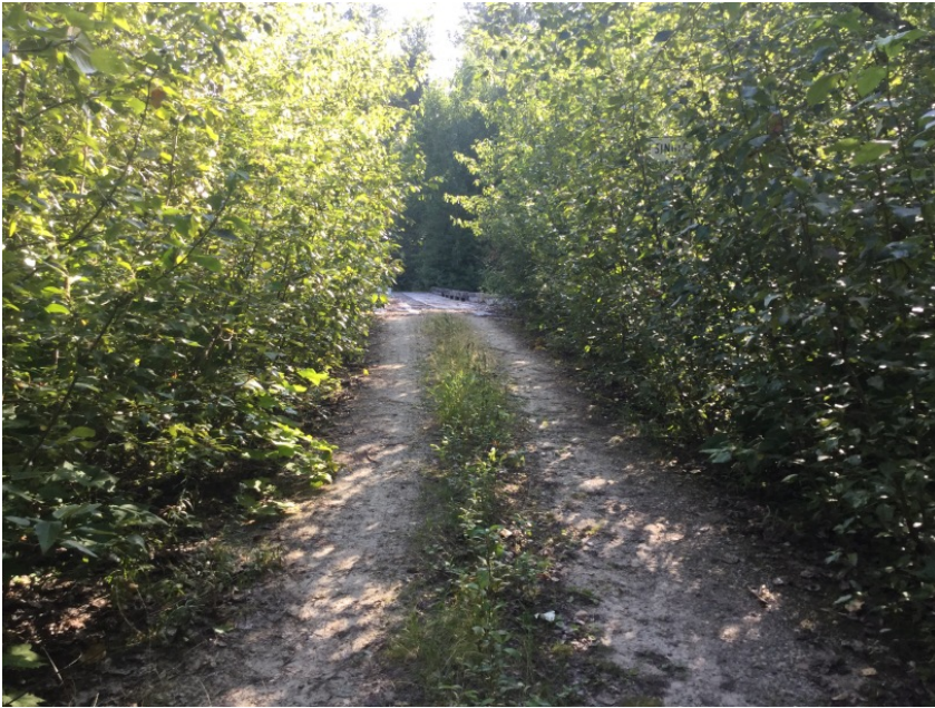
Left Approach Facing Bridge
