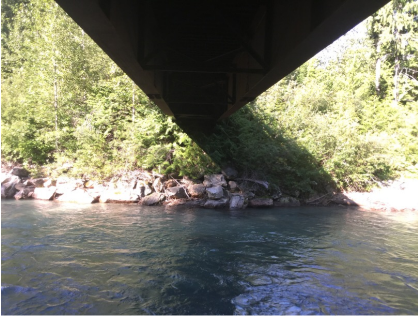
Left Bank Abutment
