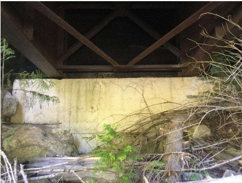
Right Bank Abutment
